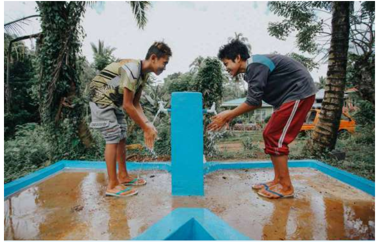
Over 100 households and 1,600 schoolchildren now have better access to safe water in South Upi, Maguindanao, Philippines, thanks to a joint project by the International Labour Organization and the Government of Japan.
